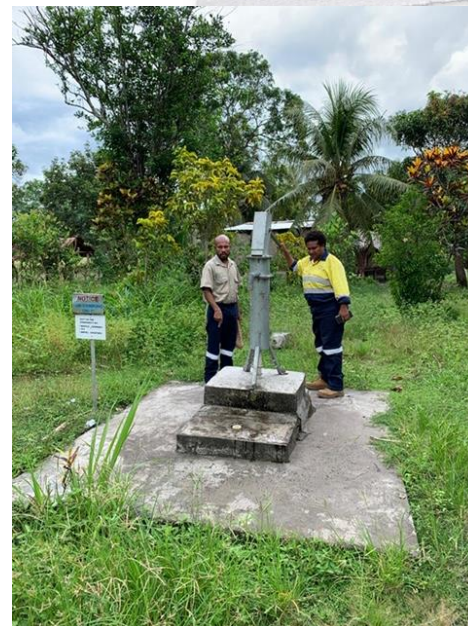
Figure 11. Newly installed clean water pump
